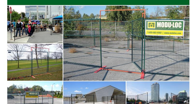
Modu-Loc fence systems include pedestrian and vehicle access gates. Our gates can be placed anywhere in the fence line, allowing for effective control.
